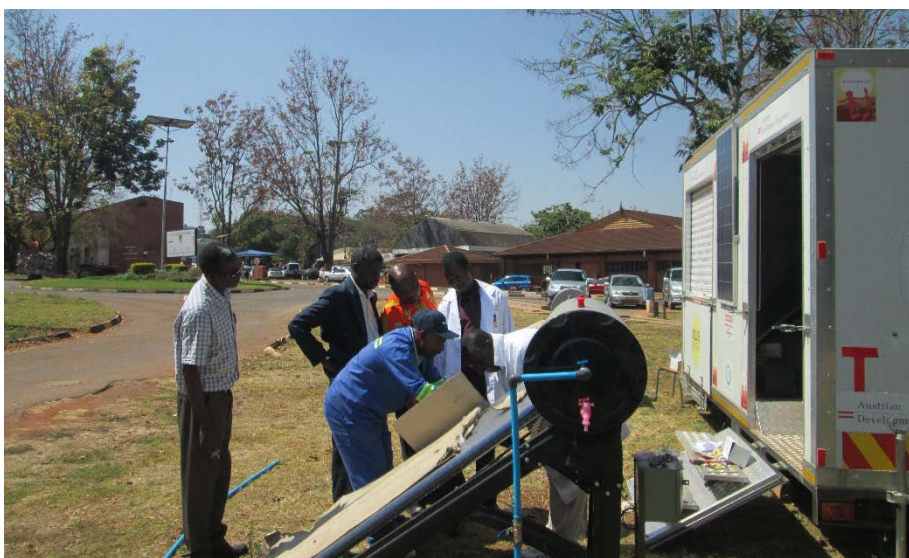
Fig. 2 – Installation of the solar thermal testing systems
