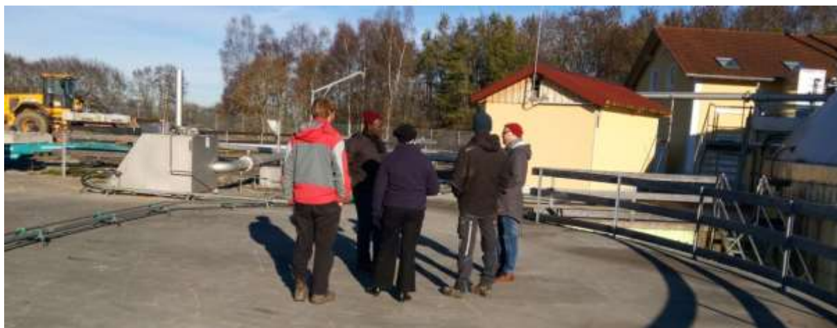
Standing on a biomass digester in Zellerfeld
